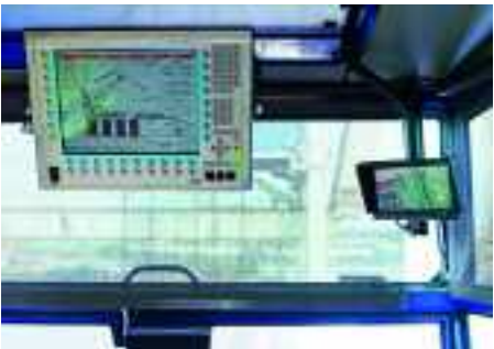
Visualisation of crane data via Crane Management System
